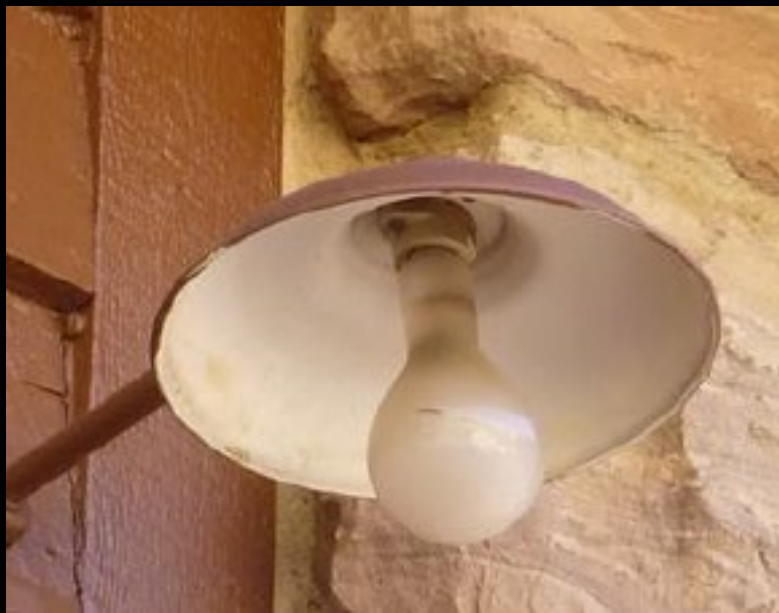
Historic light fixtures at the Maintenance yard have shallow shields; replacing large incandescent bulbs with short LED lamps to maintain historic integrity
